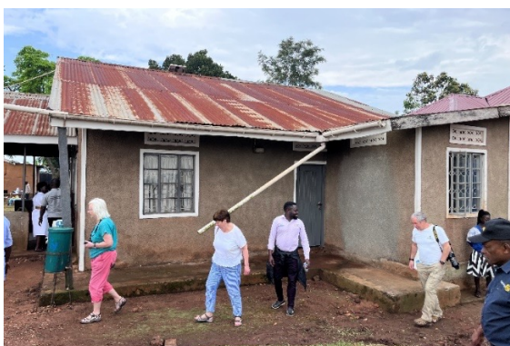
The existing maternity ward
