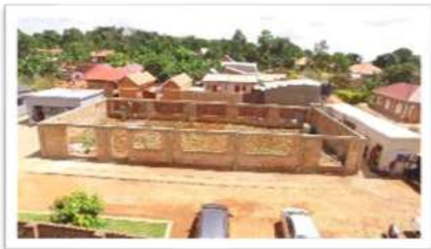
The current position of the building project
