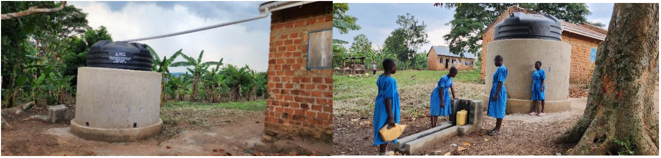
Mwererwe Primary School Latrines and Water Tank. Funded by a grant from the Hilden Charitable Fund.
